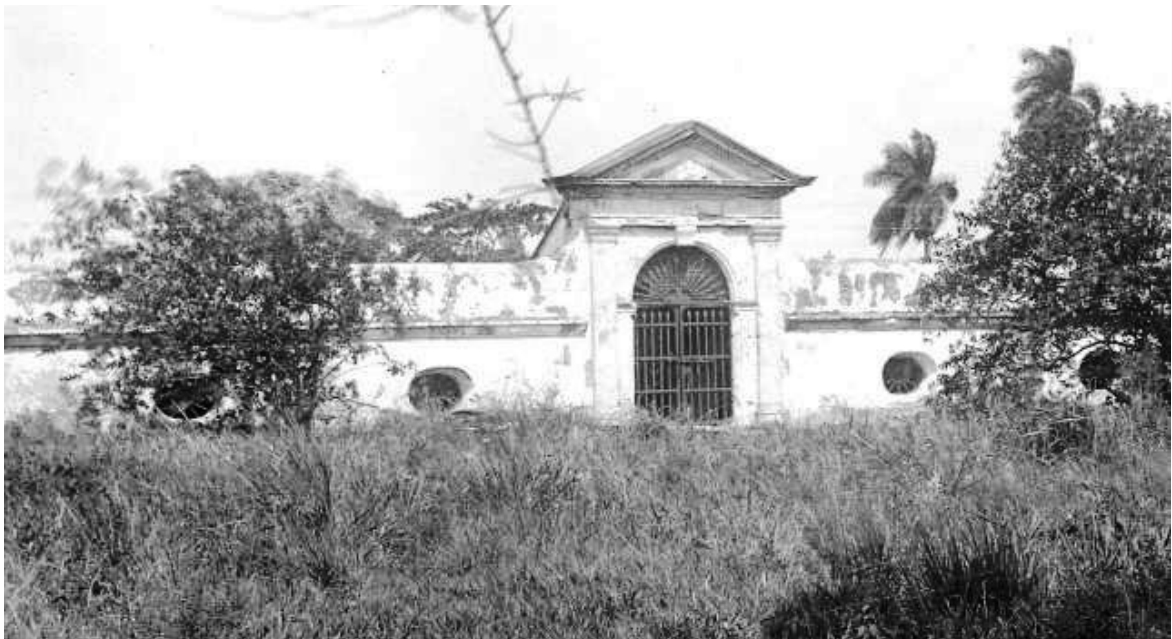
Figure 7. Principal Facade of the Fernando II Aqueduct (Photo taken in 1926)
