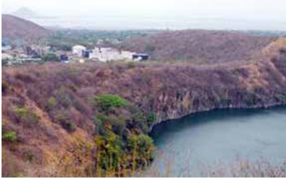
Figure 2.4 The Refinery on the North Bank of the Asososca Lagoon
