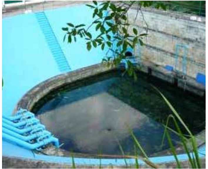
Figure 9. Vento Springs water intake today
