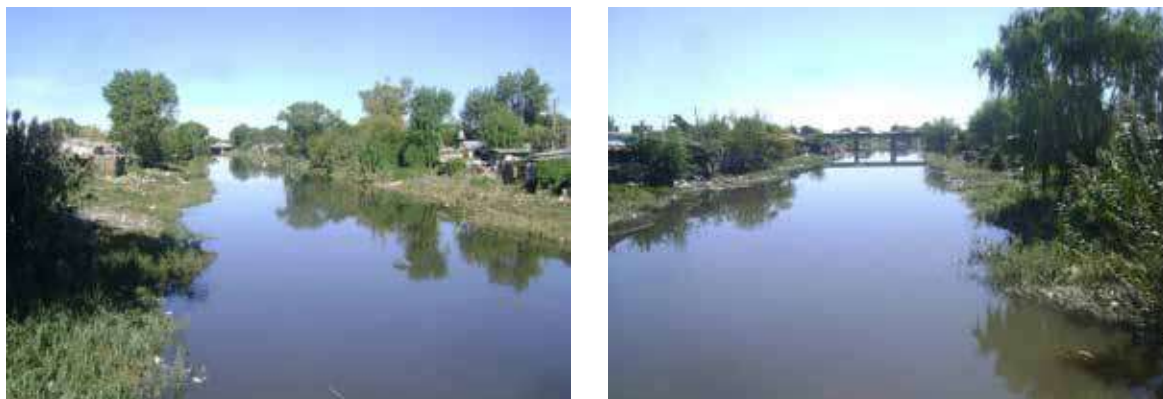
Figure 14. Structural vulnerability in the discharge of the Gato Stream – La Plata
