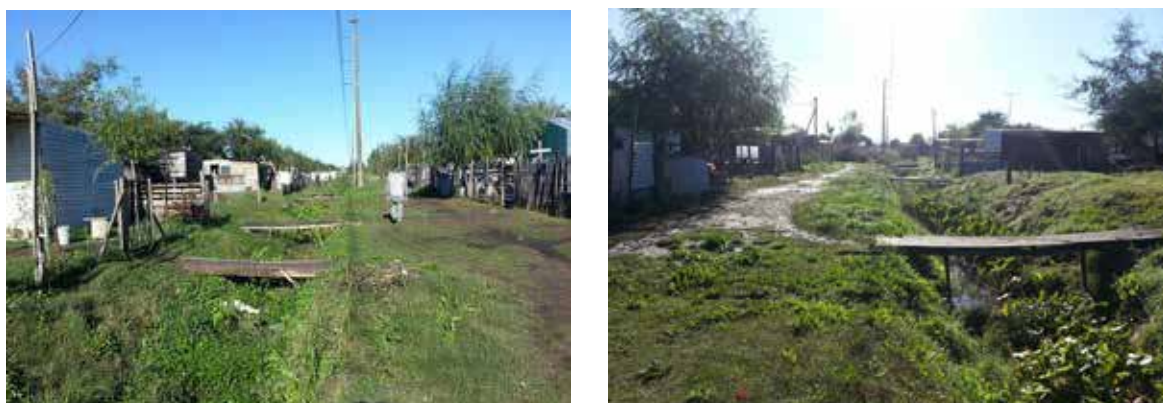
Figure 15. Structural vulnerability in the discharge of the Maldonado Stream – La Plata
