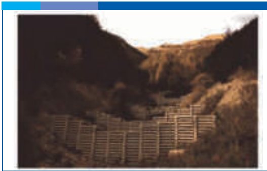
FIG. 25. Check-dams Constructed with Pre-fabricated Concrete Joists
