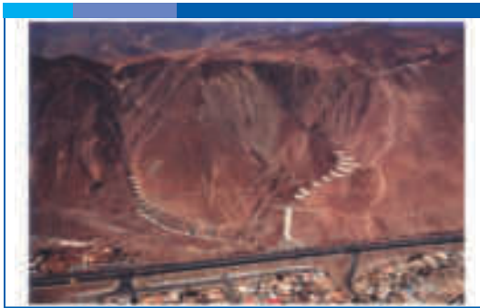
FIG. 26. Panoramic View of Chek-dams Built in Ravines El Ancla and Baquedano, Antofagasta (MOP, 2009)
