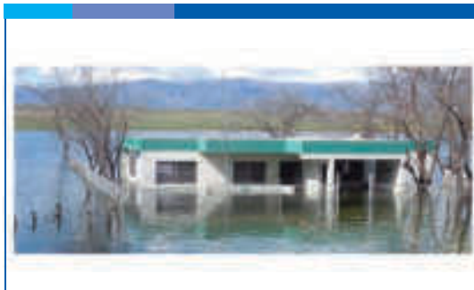
FIG. 8. Frontier Agricultural Offices Flooded by the Rising Waters of Lake Sumatra, to the West of Jimaní
