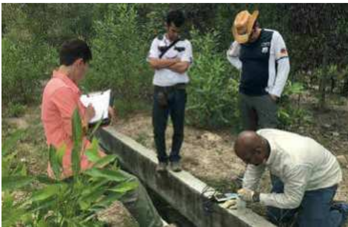
➤ PRCC. Cocabel, Wastewater Treatment Plant, Lempira, Honduras.
