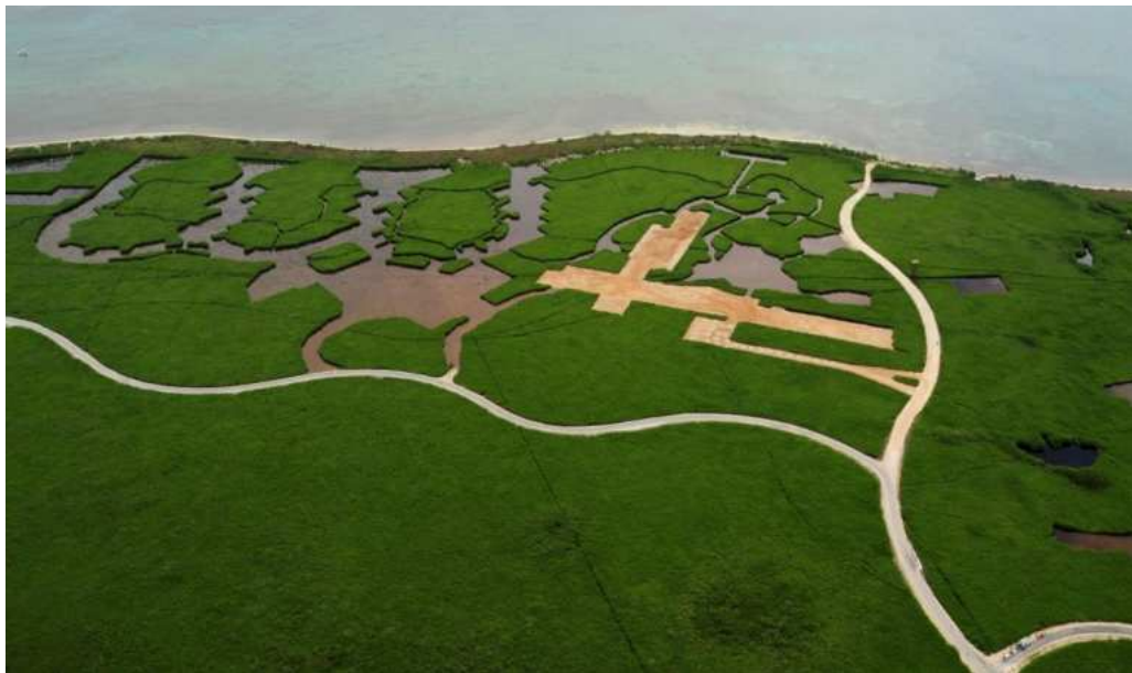
Development of tourism infrastructure in the mangrove areas of the Riviera Maya, Mexico (photo credit: CONABIO-SEMAR/Carlos Troche).
