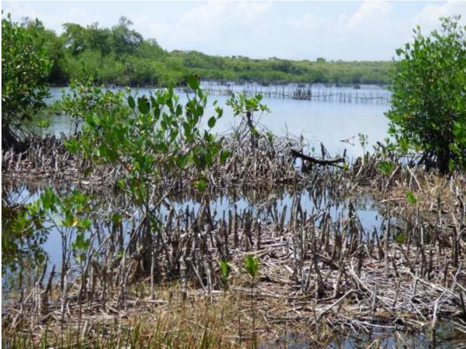
Annex 16: Wooden dam in Lagon aux Boeufs
