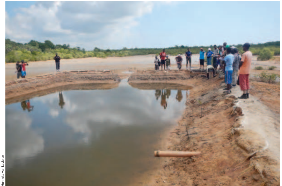
A failed aquaculture pond in Gazi Bay, Kenya.
