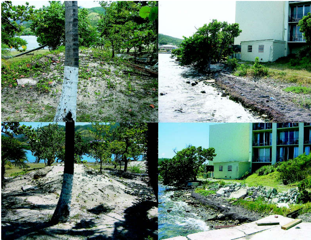
FIG. 2. a,b. Before (14 January 2002; top left) and after (20 February 2003; bottom left) photographs of habitat disturbance within unit V where Ameiva polops was formerly present. Concrete rubble now covers the site where an adult was seen near the largest shrub in foreground before disturbance. 2c,d. Before (27 February 2002; top right) and after (20 February 2003; bottom right) photographs of habitat disturbance within unit M where Ameiva polops was absent during the winter 2002-2003 survey. Note the virtual elimination of ground cover and litter on the sand mound, and disturbed soil in the foreground.
