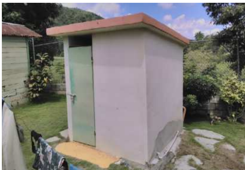
Illustration 10: Example of improved installation outside the home. Source: CORAASAN household survey.
