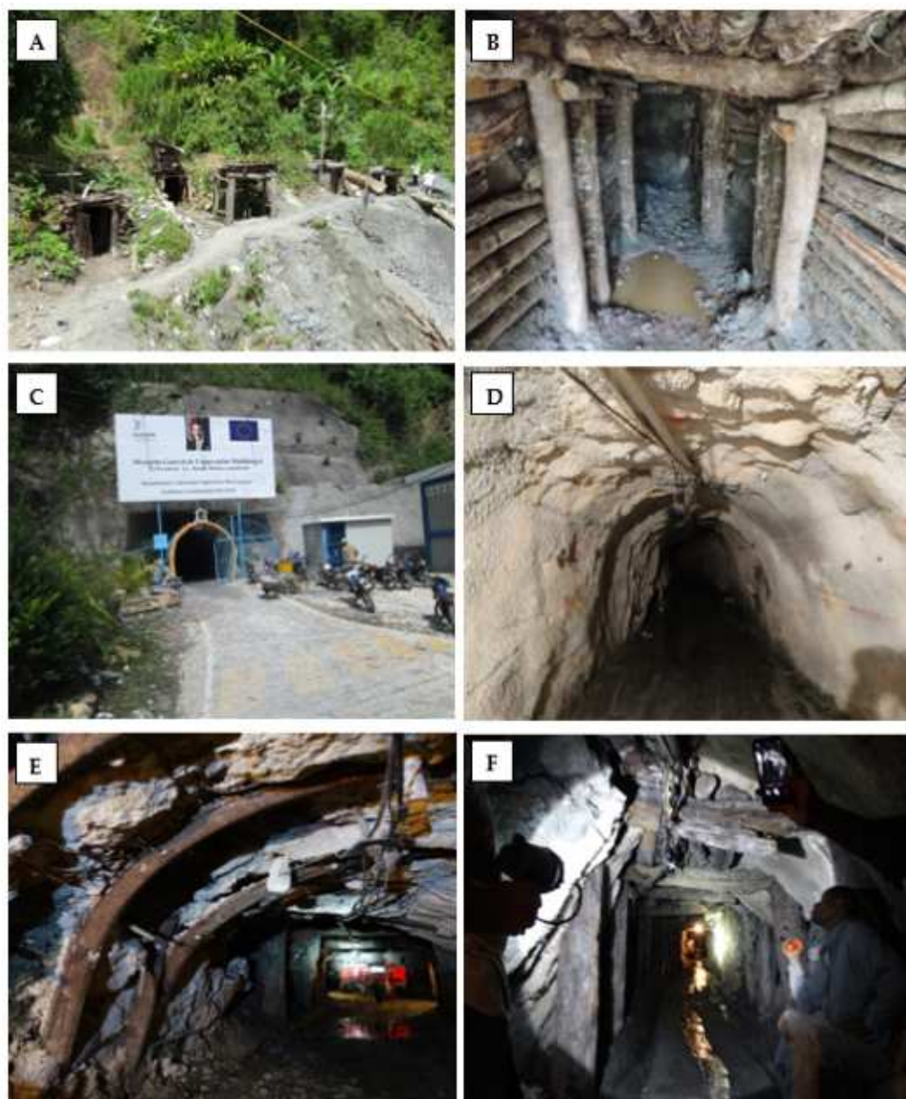
Figure 3. Mining of larimar in basaltic rocks at the Las Filipinas mine. (A,B) Shallow excavations in the slope of the hill with a primitive timber lining (as of 2013); (C,D) tunnel with steel and timber support and concrete rendering (as of 2016); (E,F) tunnel as of 2020; Photographs were taken by L. Natkaniec-Nowak and K. Broda.
