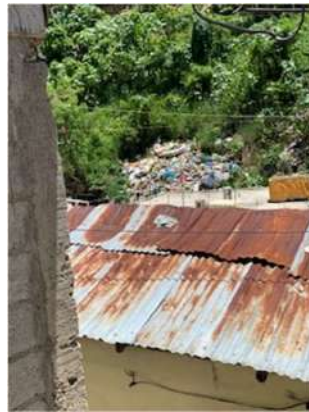
Photo 6-4: Zinc-Roofed Housing in the Area of Influence of the Project
