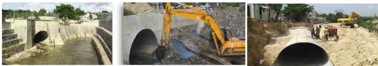
Photo 1-3: Canal Buenos Aires Works
