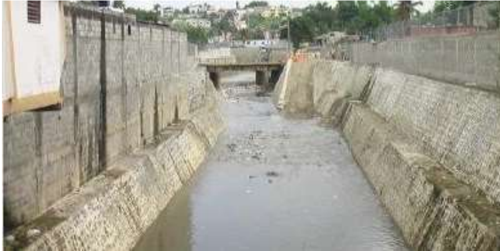
Photo 4-6: Re-profiling of the Guajimía Canal in the Section from 400 m Upstream of the Guajimía-Buenos Aires confluence to the 6 de Noviembre Highway Bridge that was executed as part of Phase I of the Project
