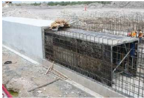
Figure 3-1: Reinforced Concrete Box Culvert
