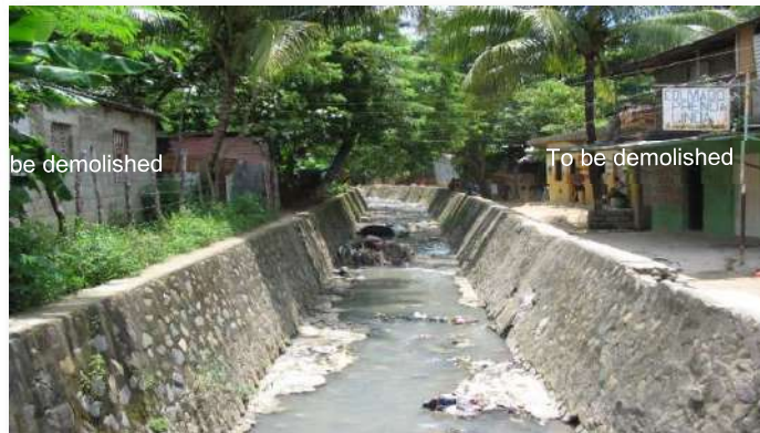
Photo 4-2: Buildings on the Banks of Canal needed to be Demolished
