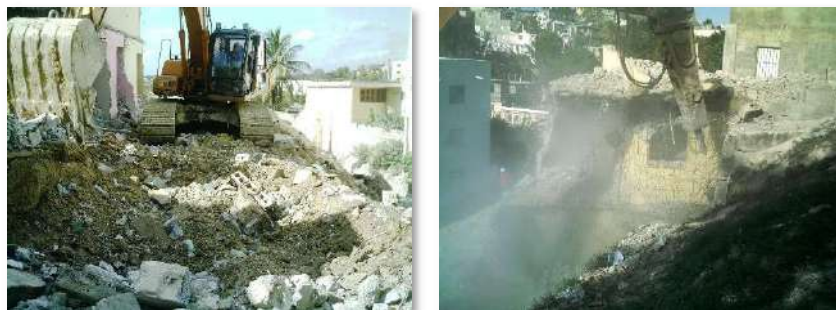
Photo 4-3: Demolition of Houses using Powered Mobile Plant in Phase I of the Project
