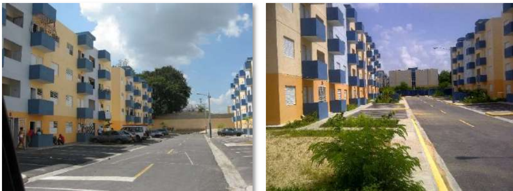
Photo 4-1: Residential units Constructed for Phase I of the Project
