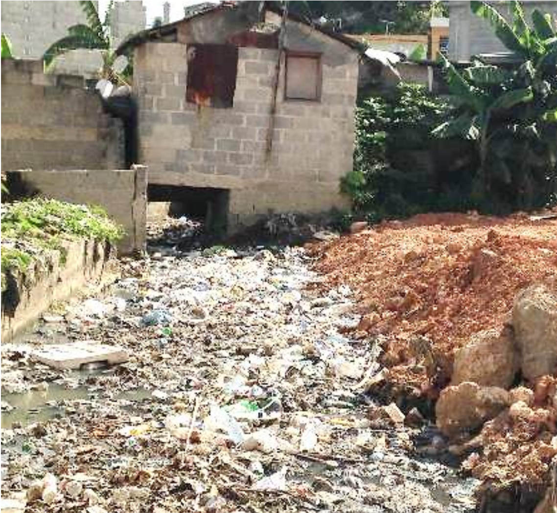
Figure 1.1: Solid Waste Accumulation in Channelized Creek in Los Platanitos
