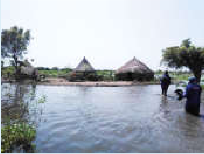
Figure Box 9.2.1 | Indigenous earth walls ( hayit ) built by Indigenous people in Akobo, Jonglei Region, South Sudan, to protect their houses and infrastructure from the worst flood in 25 years that occurred in 2019. The wall is 1–2 m high. Photo credit: Laurent-Charles Tremblay-Levesque.
