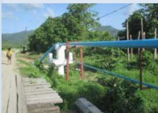
Pipeline Raised Above Flood Level
