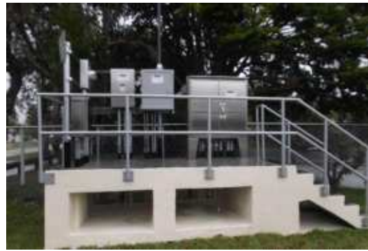
Figure 3. Elevate Critical Structures
