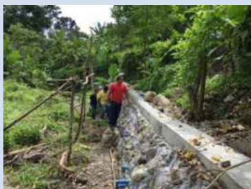
Concrete encased pipeline for erosion protection
