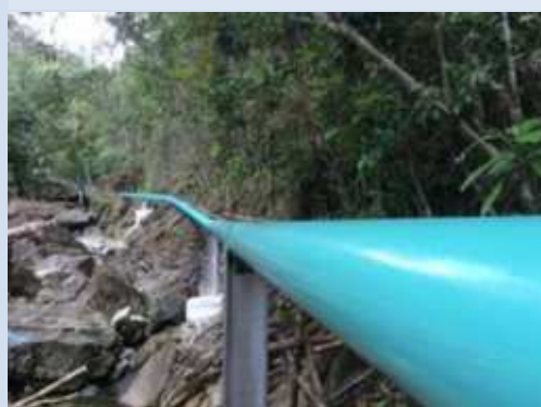
Realigned Pipeline Along Stable Slope
