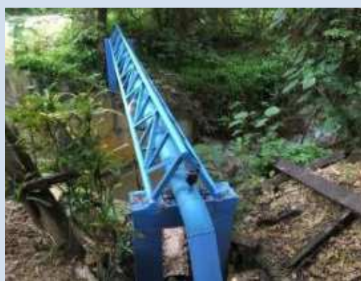
Hardened Pipeline River Crossing
