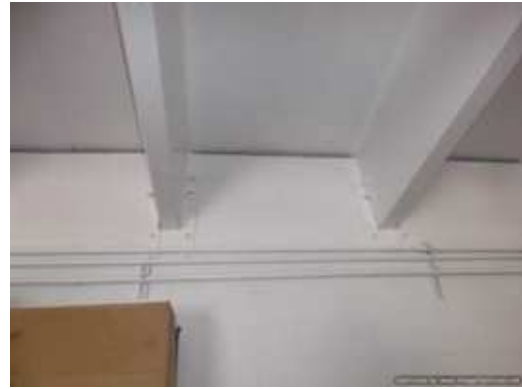
Figure 3. Tee roof beam brackets added to resist wind uplift forces.
