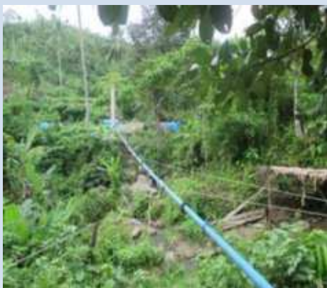
Cable hanging of pipeline above river
