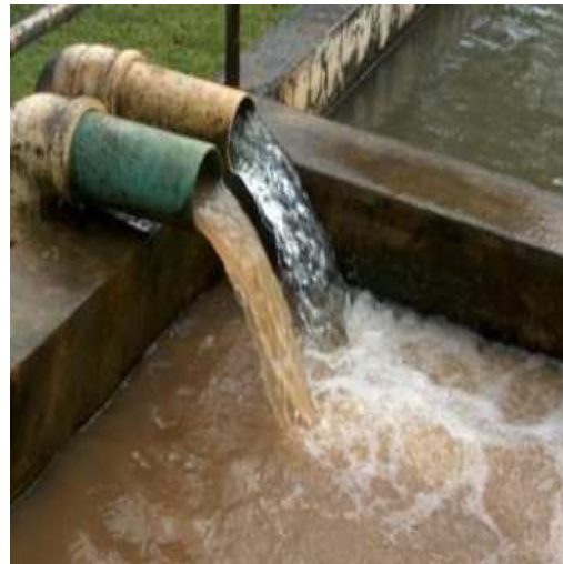
Figure 2. Water discharge to treatment plant from a poorly managed watershed (left intake)
