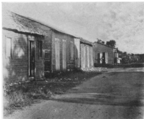
FIG. 8—The main street of a typical town of the Dominican Republic. The sides of the houses are made from boards cut from the highly utilizable palm.
