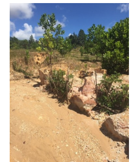
Live check dams using sustainable forest materials
