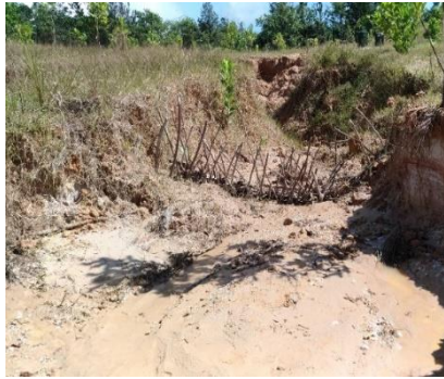
Photo 1: Live check dams installed to reduce erosion.
