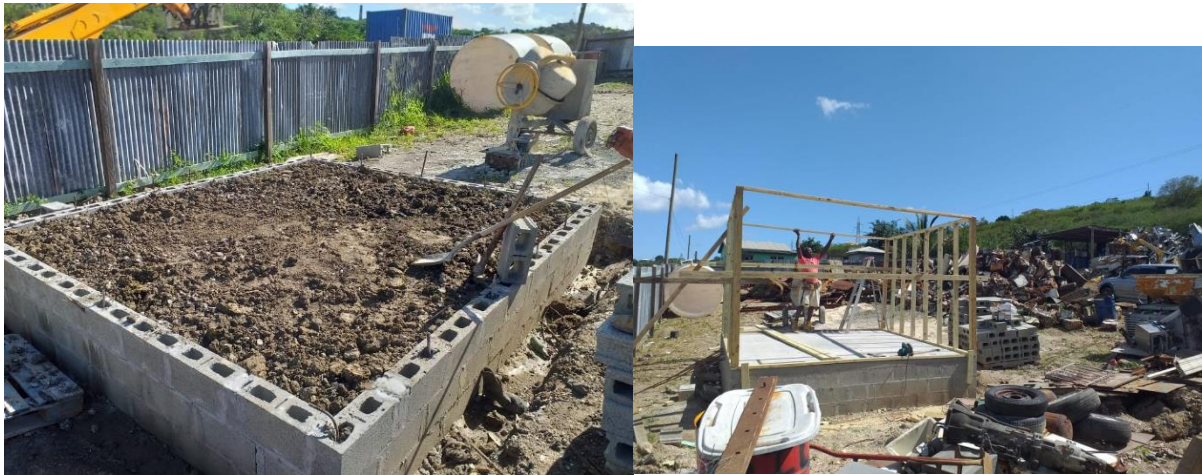
Photo 2. Construction of wire stripping center to house equipment
