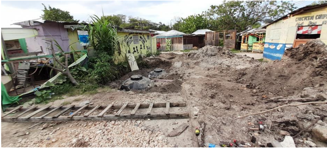
Photo 6. Septic tank installation at Discovery Bay Fisherman Beach
