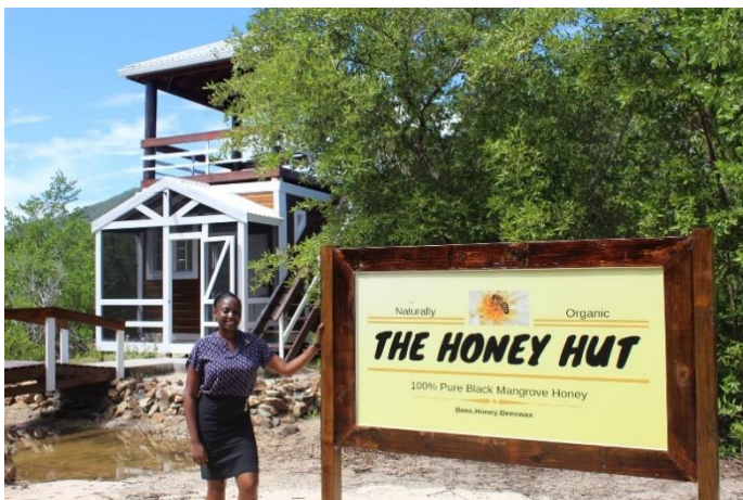
Photo 4. Constructed honey facility on Union Island, St Vincent and the Grenadines
