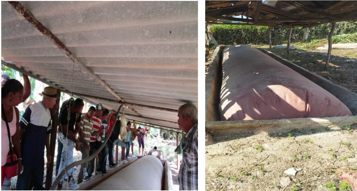
Photo 4. A demonstration training workshop for the installation of a 10 cubic meter geomembrane tubular biodigester on the farm of a producer.
