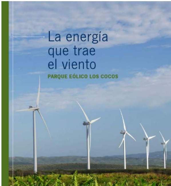
Figure 9-3. wind energy farm in the Dominican Republic
