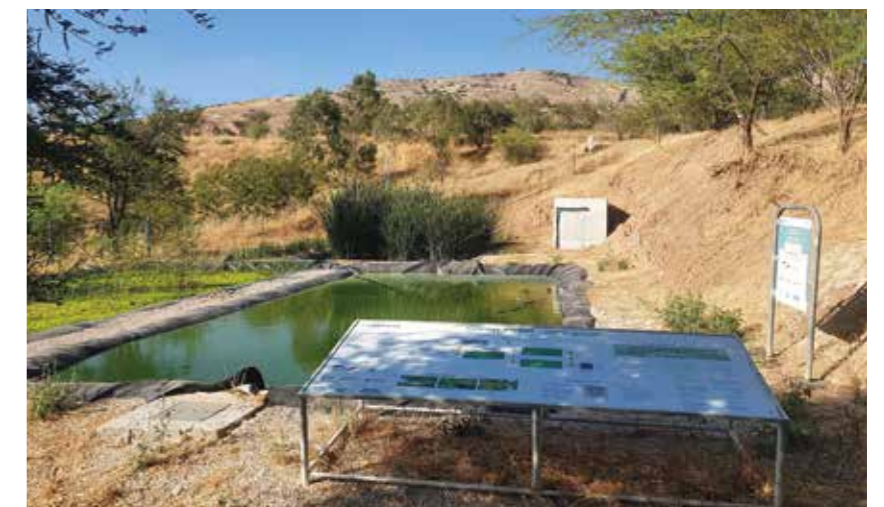
The Green Filter built by the GNF and EcoPeace Middle East in Jordan EcoPark.
