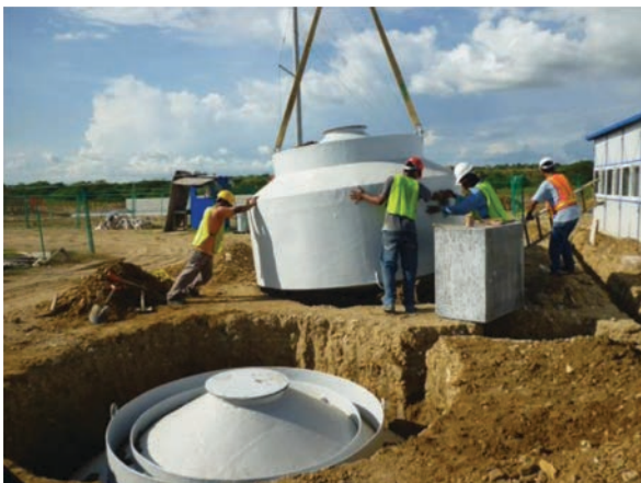
Figure 4: Using prefabricated fiber-reinforced plastic or monolithic concrete (around 500 people for this office building in Miramar) the installation time can be reduced to 3 days.
