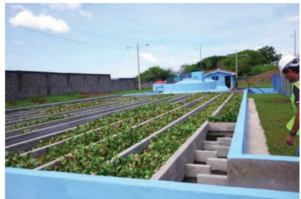
Figure 3: Additional perspectives on the Nature-Based Solution for wastewater treatment of the new housing developments in Nicaragua.
