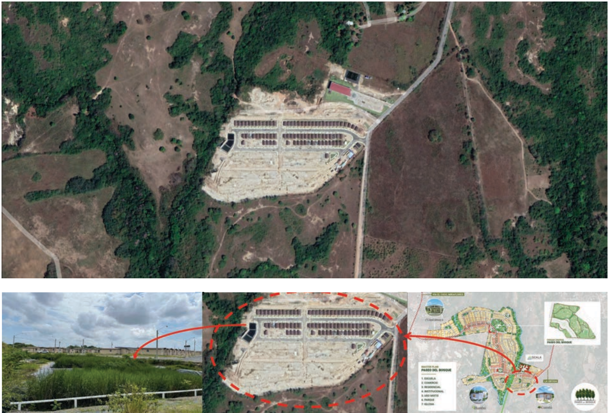
Figure 3: The Nature-Based Solution for wastewater treatment in Penonome is part of a larger housing development that will be built in the coming years. Further treatment systems will be added as construction progresses.
