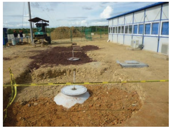
Figure 4: Using prefabricated fiber-reinforced plastic or monolithic concrete (around 500 people for this office building in Miramar) the installation time can be reduced to 3 days.
