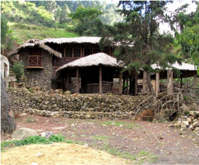
Photo 6. The partially-constructed restaurant located just outside of El Convento.
