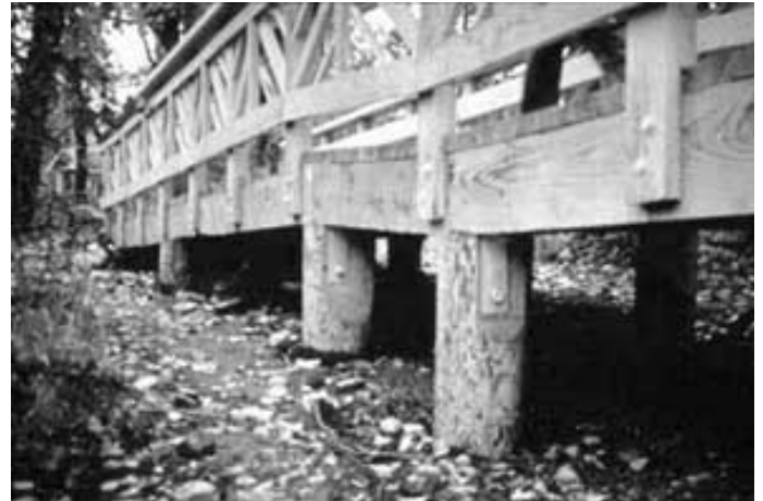
Photo 2 – Wood poles used as the pylon to support the boardwalk trail.
