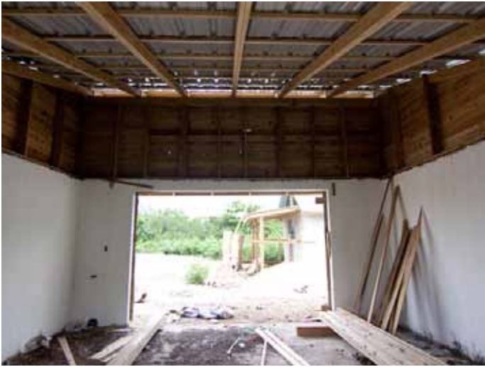
Photo 15 – Inside view of the 3 attached units. These separate spaces could be used for a small gift shop and visitor information center.
