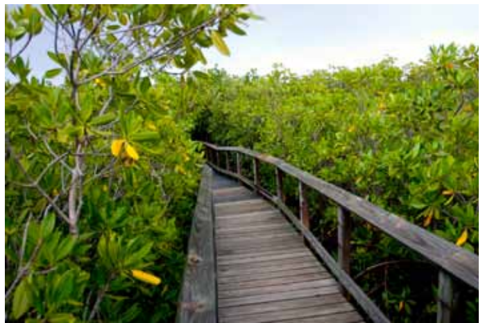
Photo 10 – Close view from the boardwalk platform, notice the handrails.
