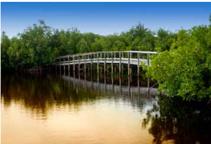
Photo 9 – Distance view of boardwalk in the mangrove forest.
