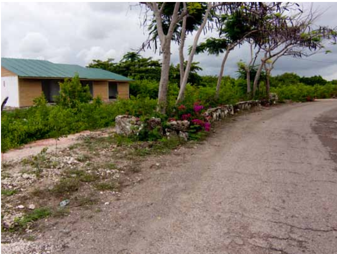
Photo 13 – Access road leading to Refuge entrance. The existing cement structures that are being rebuilt are on left. A small bus (Coaster) parking area could be developed along the road at lower left of this photo.
