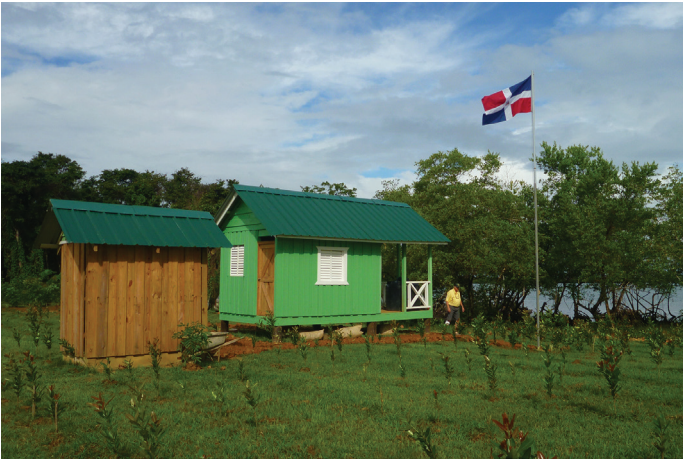
Photo 1 – Ministry of Environment guard station at La Gina. This is the only infrastructure in the Refuge.
