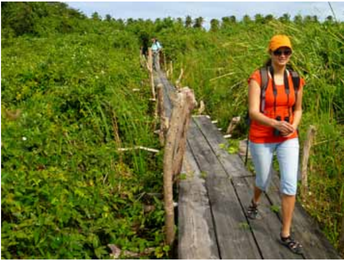
Photo 9. Boardwalk leading from Limón Beach to the lagoon. This is a safety hazard to visitors.
