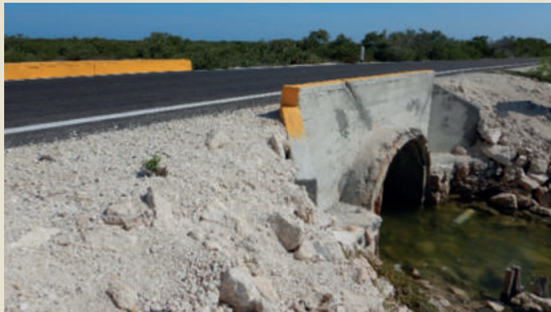
Culvert blocked with debris
