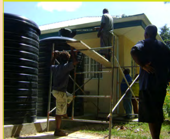
Figures 52 & 53: Caura Valley residents install a rainwater harvesting system. January 2013. Credit: CANARI
